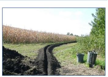
Figure 3. Construction of Bear Creek seepage lateral in the riparian zone (Jaynes et al., ADMC website).
