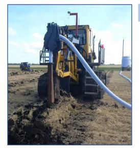
Figure 1. Installation of tile drainage on an agricultural field.
