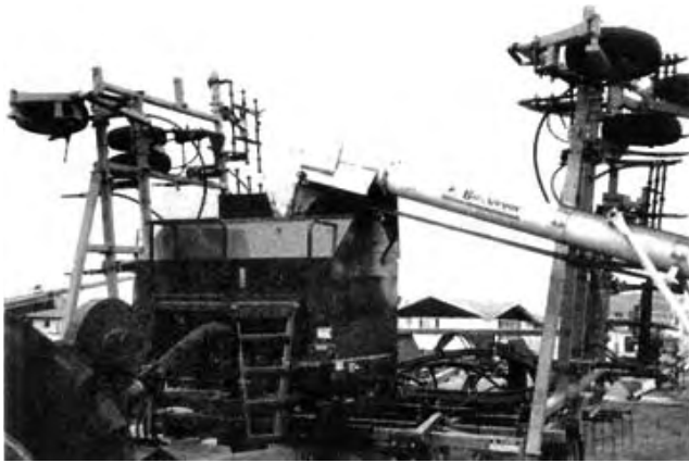
FIGURE 5. Filling with a Conveyor Auger.
