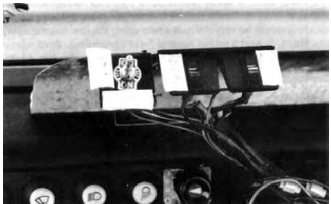
FIGURE 8. Injector and Sprayer Control Panel (Note: Labels Added by PAMI).
