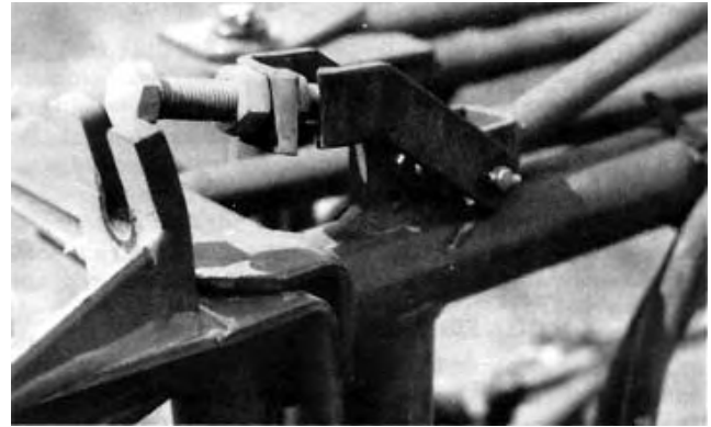
FIGURE 19. Failed Boom Lock Bracket.
