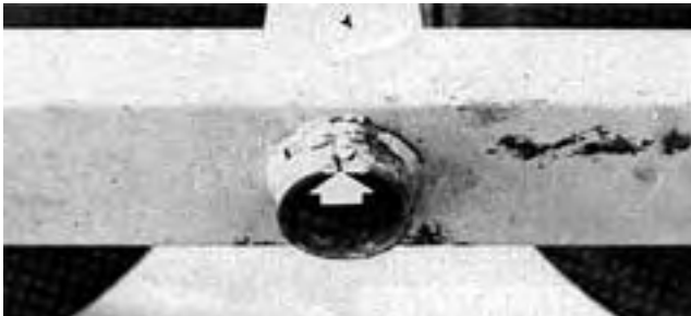
Figure 22. Cracked Rocker Arm Bushing.
