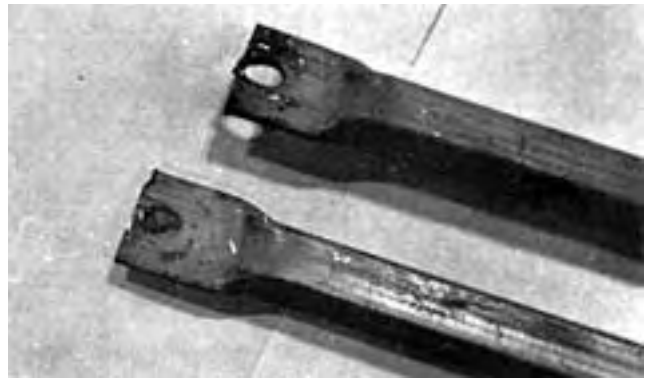
Figure 22. Worn Radius Brace Holes.
