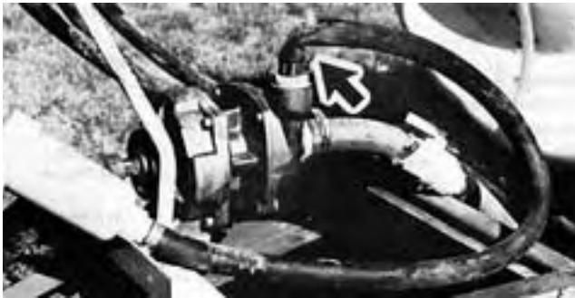
FIGURE 17. Buckled Pump Outlet Hose.
