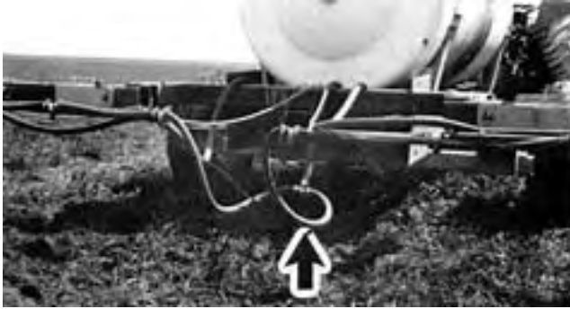
FIGURE 16. Sagging Middle Boom Inlet Hoses.
