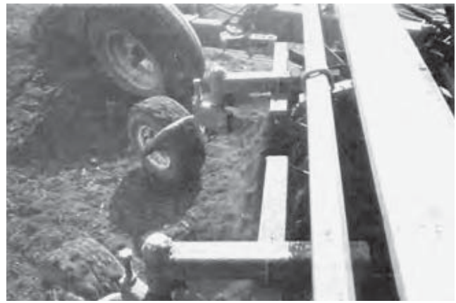
FIGURE 3. Operating in Wet Loam Soil.
