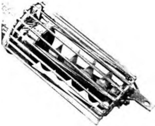
FIGURE 7. Removable Inlet Safety Guard.
