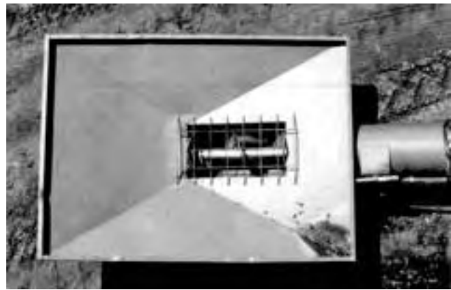
FIGURE 4. Inlet hopper and safety guard.
