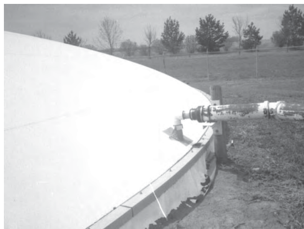
Another manure storage covering method.
