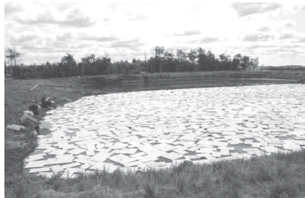
Floats in place on a liquid cell - a method that does not work.
