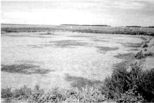
FIGURE 5. Sinkage of Unsupported Cover.
