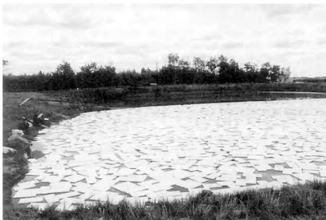
FIGURE 2. Floats in Place on Liquid Cell.
