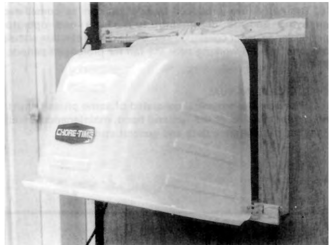
FIGURE 4. Hood on Fan Discharge.
