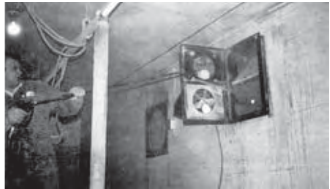
FIGURE 4. Washing with a Pressure Washer.
