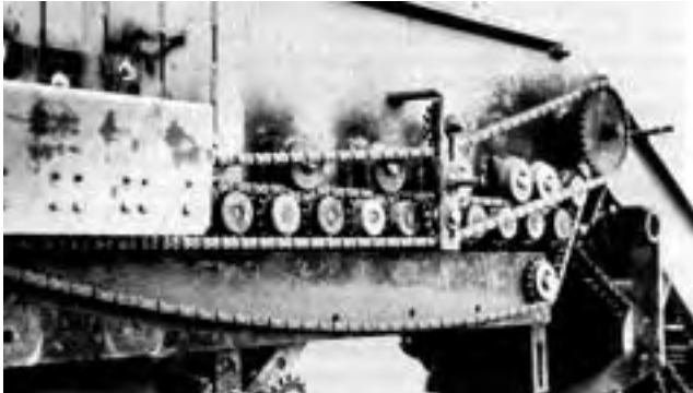
FIGURE 8. Modified Clod Table Drive Assembly.
