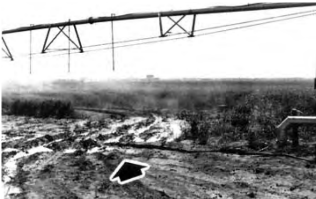
FIGURE 13. Inconvenient Control Panel Access due to High Applications Near the Pivot.
