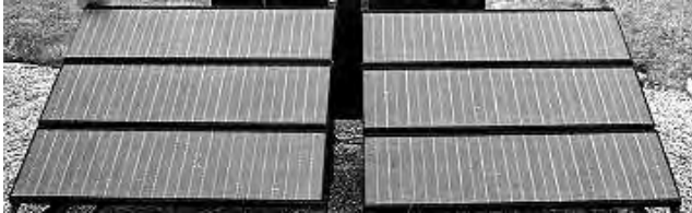
Figure 1. Kelln 6 Module Water System (Parallel/Series).
