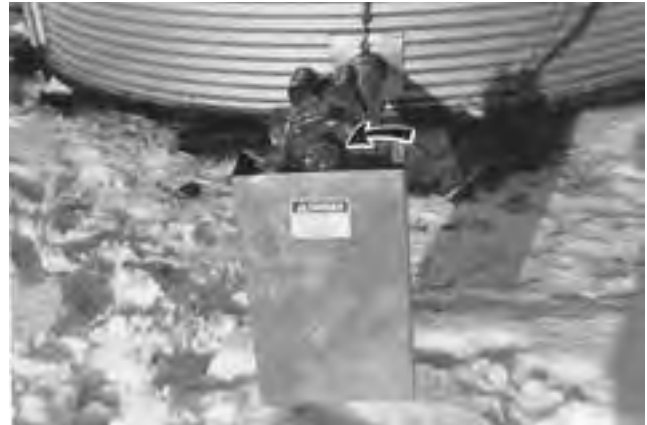
FIGURE 11. Exposed Discharge Auger Drive.
