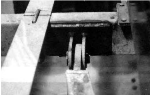
FIGURE 7. Repaired Hitch Mount Lug.
