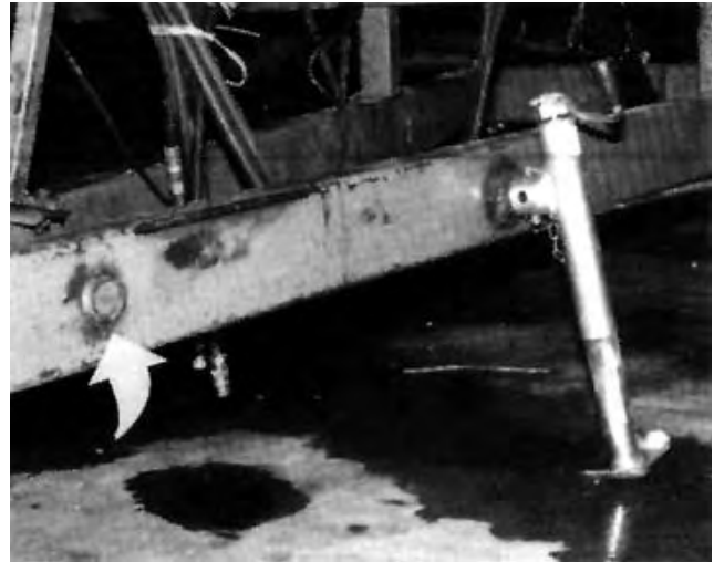
FIGURE 5. Relocated Implement Jack (arrow indicates original position which allowed interference with the tractor wheel).
