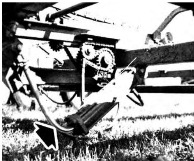
Figure 7. Pickup Fork Cylinder Shaft Failure.
