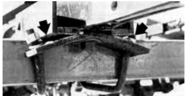
FIGURE 12. Weld Failure and Bent Rod Shank Holder.
