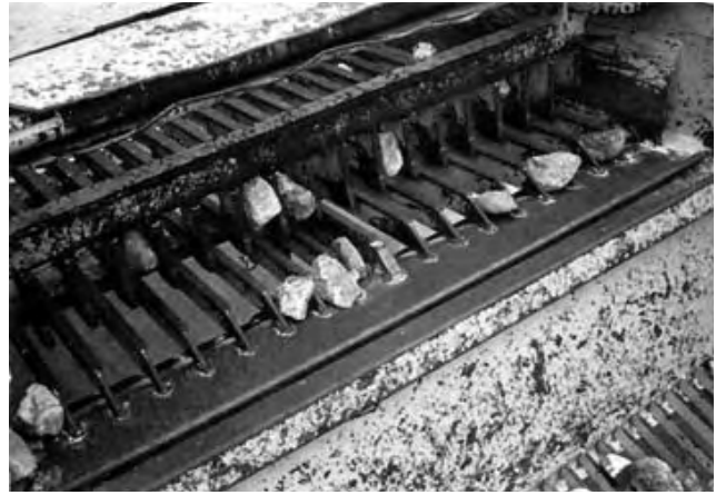
FIGURE 3. Small Rocks Jammed in the Grate.
