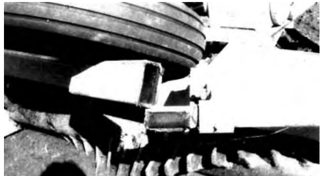
FIGURE 5. Weld Failures on Long Stabilizer Arm.
