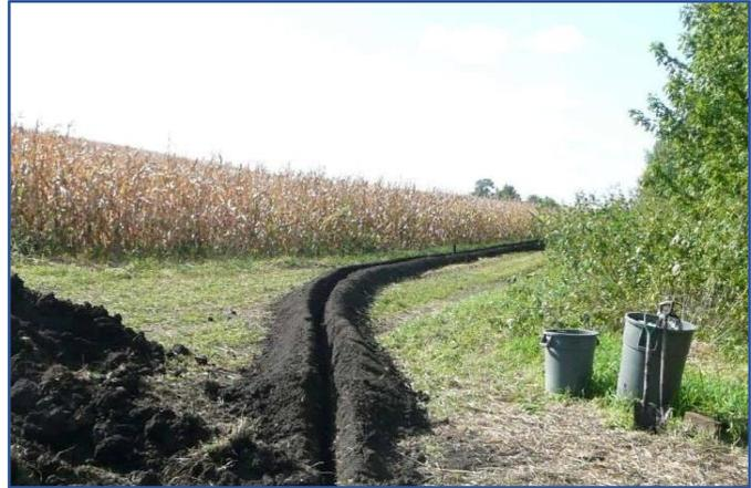
Figure 3. Construction of Bear Creek seepage lateral in the riparian zone (Jaynes et al., ADMC website).
