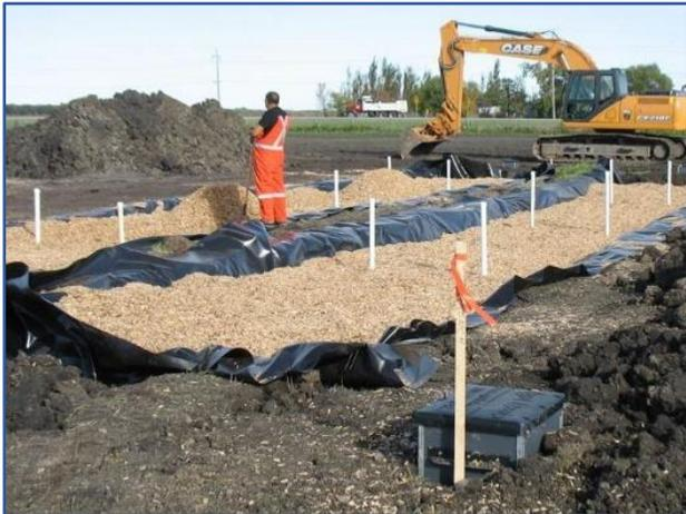
Figure 1. Construction of woodchip bioreactor at the Morden Research Station (Agriculture and Agri-Food Canada).
