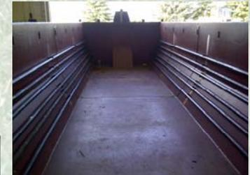
Heated glycol is pumped through a series of pipes to help maintain mesophilic temperatures in the reactor. The shipping containers also have forced air heating.
