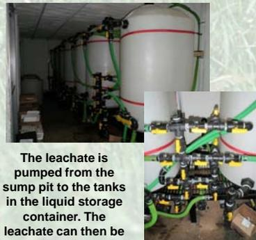
The leachate is pumped from the sump pit to the tanks in the liquid storage container. The leachate can then be stored or redistributed to the reactors.
