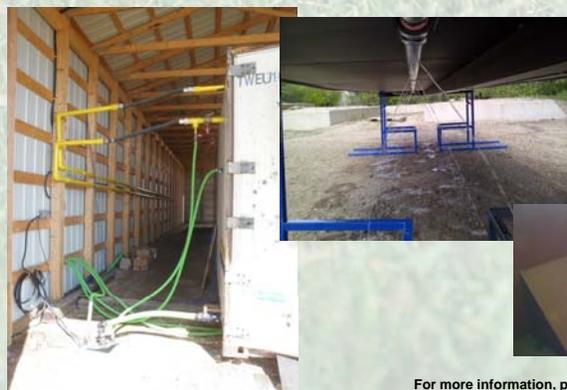
Under the lid of the reactor, perforated pipes re-distribute the leachate inside the reactor. Drains in the reactor lead to the sump pit for collection.
