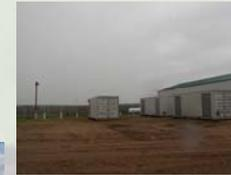
The ISO containers contain the control, gas, and liquid systems. The shed houses the reactors.
