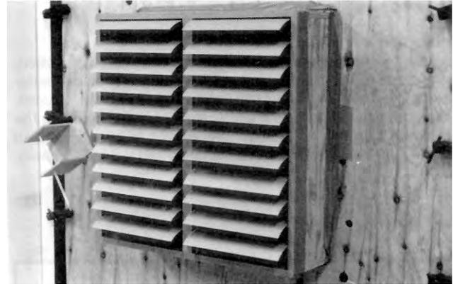
FIGURE 4. Louvres Located on Fan Discharge.
