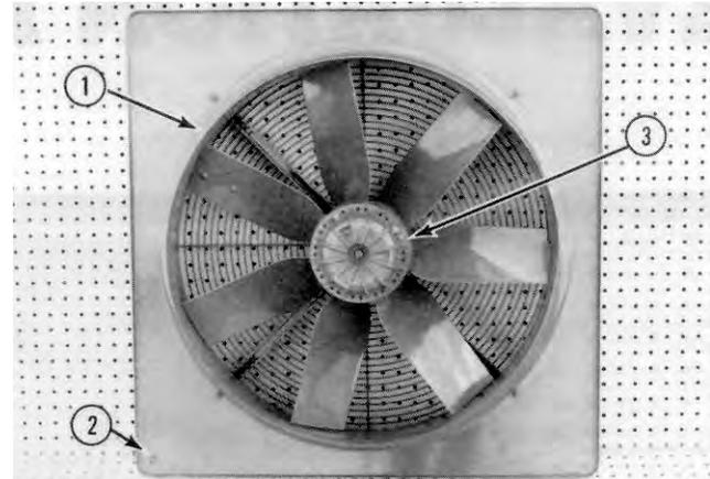
FIGURE 1. Ziehl-Abegg Model 562-6 Fan: (1) Mounting Flange, (2) Inlet Bell, (3) External Rotor & Hub Assembly.
