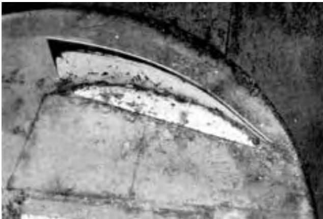
FIGURE 3. Fin on Tub Floor Repositioned.
