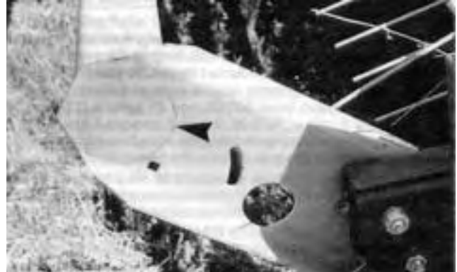
FIGURE 6. Cracks in Push Bar Mount Before Failure.
