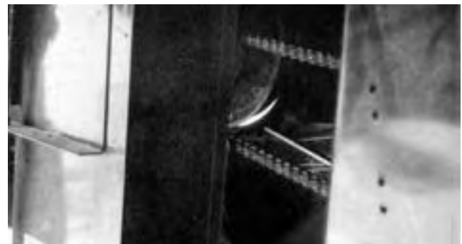
FIGURE 22. Damaged Sheet Metal on Grain Elevator.
