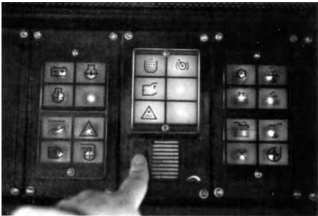
FIGURE 16. Warning Monitors in Ceiling Console.
