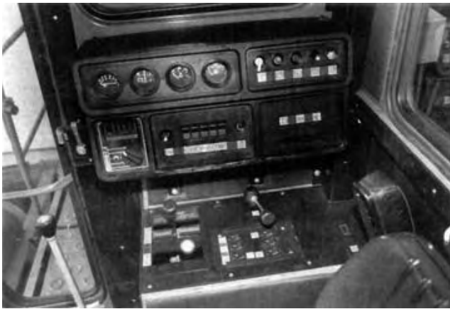
FIGURE 15. Instruments to Right of Operator.
