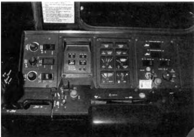
FIGURE 16. Instrument Panel to Right of Operator.
