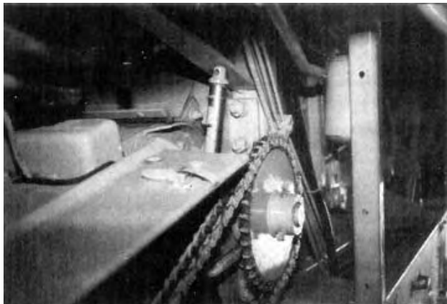
FIGURE 18. Feeder House Locking Pins Contacting Frame.
