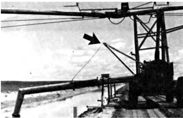
FIGURE 17. Winch for Rainger Intake Float Level Adjustment.
