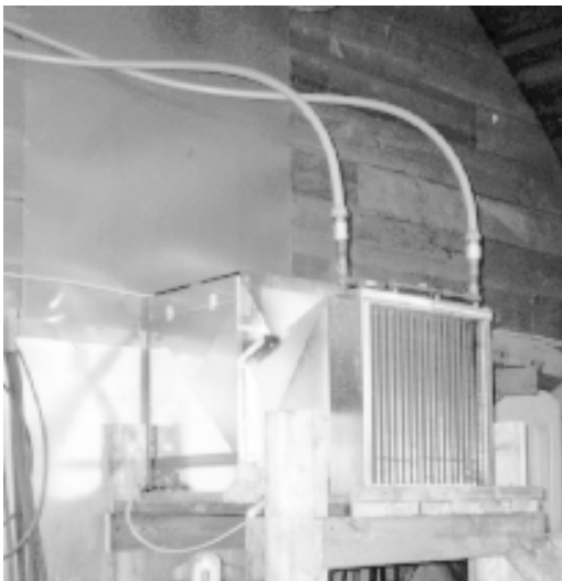
A space heater built from a radiator and fan.
