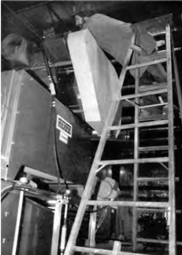
FIGURE 5. Adjusting Aspirator Controls.
